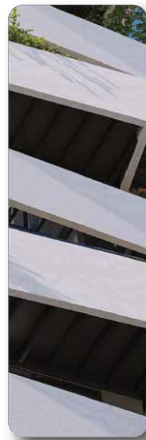
CEILING False ceiling of aluminium slats on terraces. Areas between terraces with pergolas of the same characteristics.
